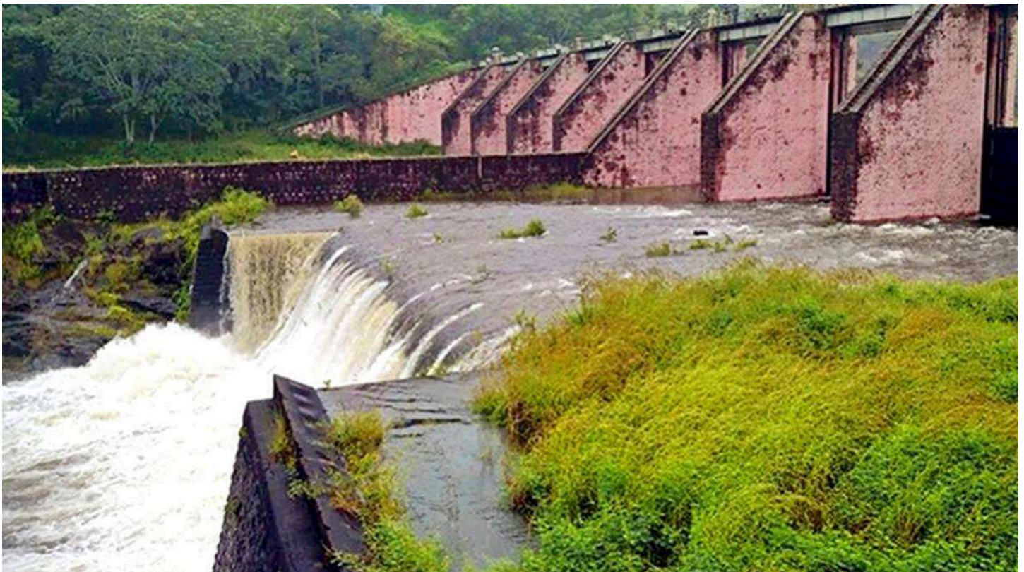
A view of the Mullaperiyar dam. | Photo Credit: The Hindu
