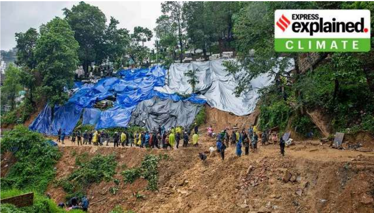
Rescue workers and officials inspect the damaged area after a stone quarry collapsed in Melthum near Aizawl, on Tuesday. (Photo: AP)
