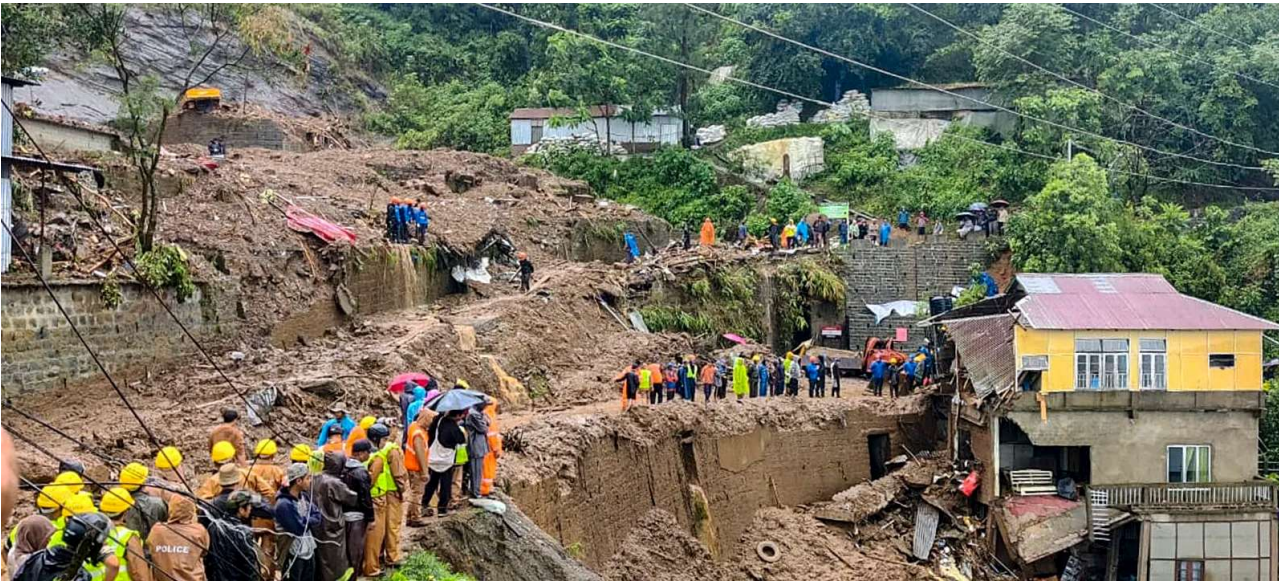
Rescue work underway after a stone quarry collapsed amid heavy rain in the aftermath of Cyclone Remal, in Aizawl district on Tuesday. (PTI Photo)
