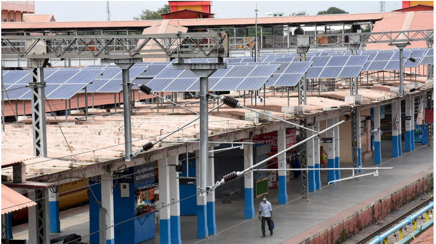
Solar panels atop a Mysuru Railway Station platform, May 8, 2022. | Photo Credit: Sriram M.A./The Hindu
