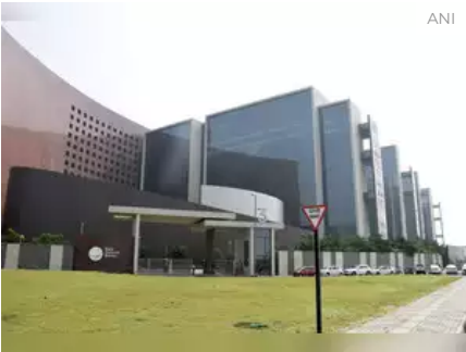
A view of the newly-constructed Surat Diamond Bourse
