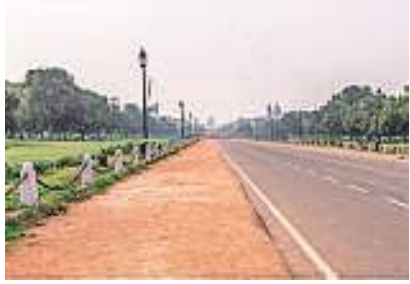
The red gravel has been replaced by sandstone
