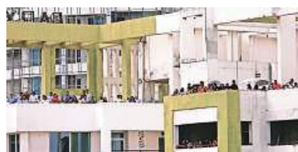
Residents watch the demolition, Sunday. Gajendra Yadav
