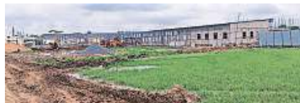
Construction at the new campus site.
