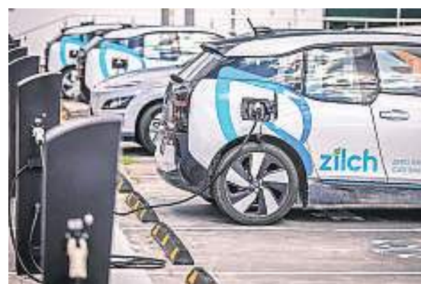
An electric vehicle charging station and car share parking in Auckland. AP
