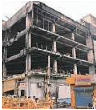
The building owner got a factory licence in 2016 which was later cancelled by the North MCD. Abhinav Saha
