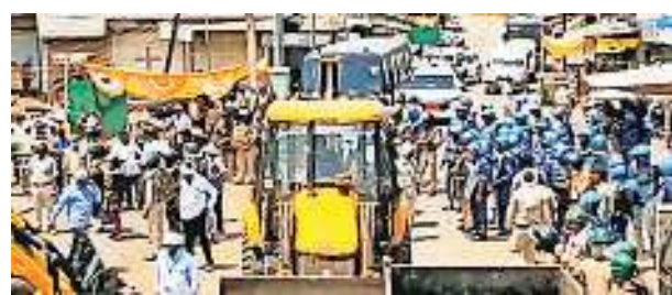
During the demolition drive in Khargone on Monday. Express
