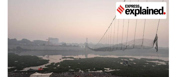
In Morbi, the vertical cables seem to have snapped entirely from the deck at one end of the bridge,
