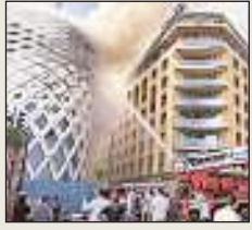
An under-construction building caught fire in Beirut on Tuesday. AP
