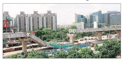
Last week, a 40-metre portion of the spine between pillars 10 and 11 of the under-construction elevated road collapsed. Gajendra Yadav
