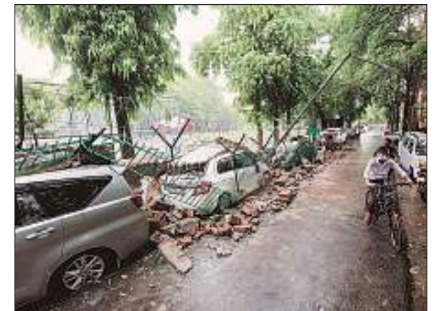
At Saket J Block, Wednesday. Seven cars were damaged in the wall collapse. Tashi Tobgyal
