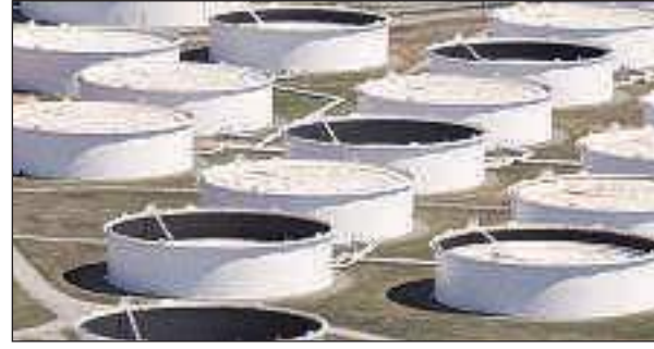
Crude oil storage tanks at the Cushing oil hub in the US. Reuters file
