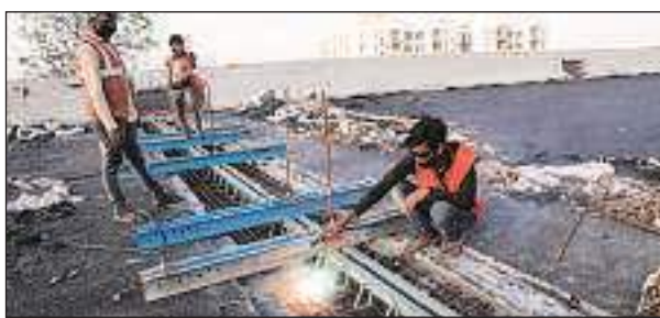
Work on Kharar-Mohali flyover restarted Tuesday. Jasbir Malhi
