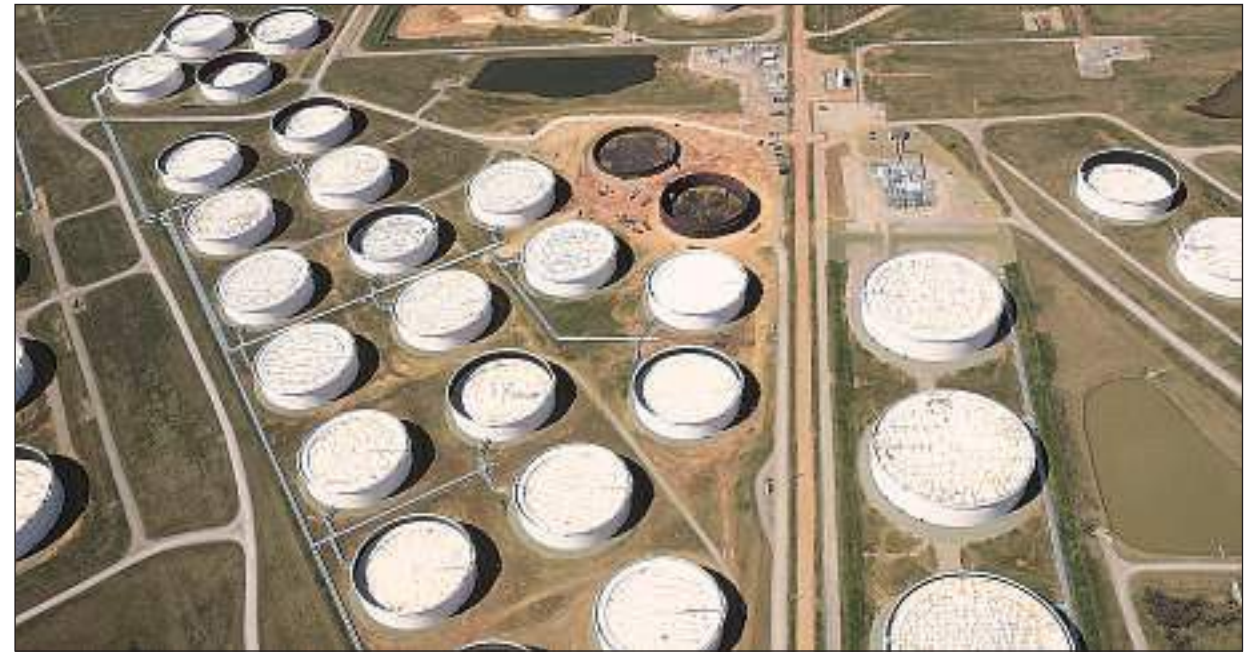
Crude oil storage tanks at the Cushing oil hub, in Oklahoma. Reuters
