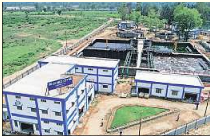
26 MLD STP, Rishikesh
