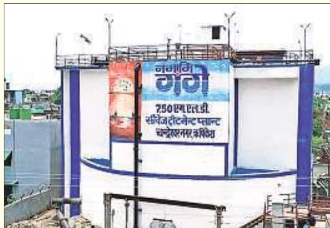
7.5 MLD STP, Muni Ki Reti, 1st 4 Story Sewage Treatment Plant
