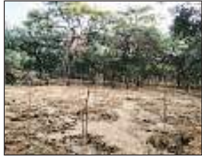
Track marks left behind by the excavators
